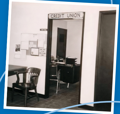
NWA Building B, 1960s
